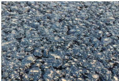
Very fresh asphalt concrete
