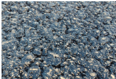
Very fresh asphalt concrete
