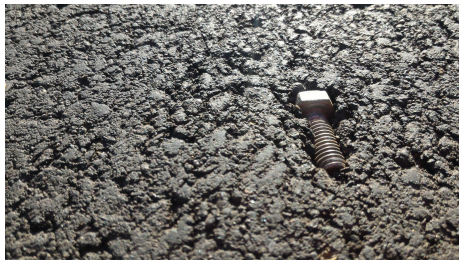
Normal asphalt concrete . . . with a bolt ☺
