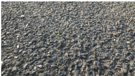
Old asphalt concrete with worn out bitumen
