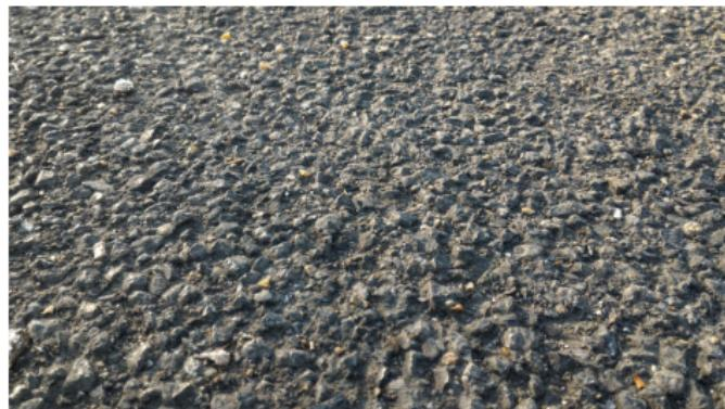
Old asphalt concrete with worn out bitumen
