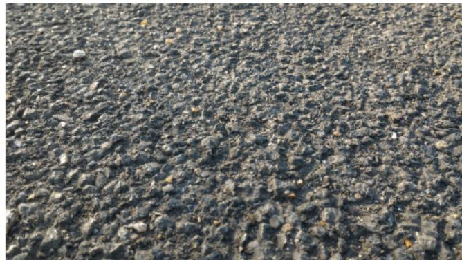
Old asphalt concrete with worn out bitumen
